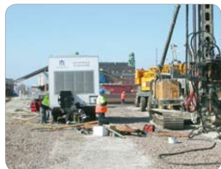
Malmö Citytunnel – Sweden Ground water screening during the construction of the City Tunnel.
