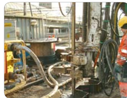
Citybanan, Stockholm – Sweden Construction of a ground water cut-off wall at the Central Station.
