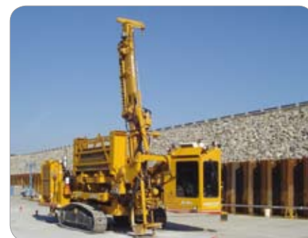
Wolf Creek Dam, Kentucky – USA Installation of grout curtain to prevent seepage.
