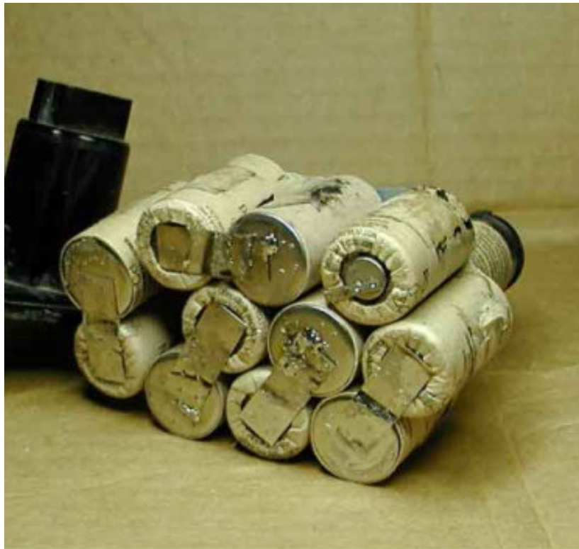
Here the new cells have been installed.
