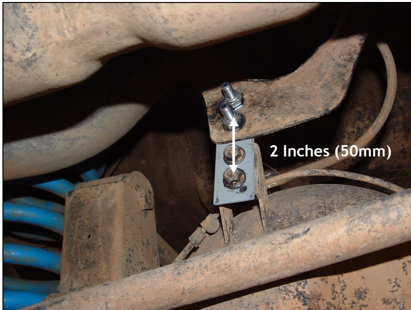
Home made bracket (2" lift), any piece of spare/scrap steel will do.
