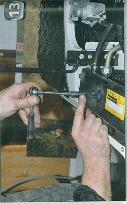
of rubber strip, foam, washers and gaskets in connection with another project and eventually came across R.H Nuttall Limited of Birmingham. Their self-adhesive foam strip was ideal for making the seal between intercooler and radiator that had been found on the original.
