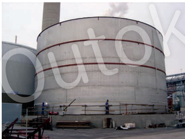
Figure 9:17. White liquor tank in duplex LDX 2101®, where corrosion resistance and strength of this grade is utilized.
