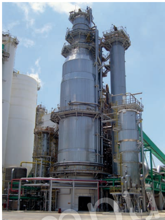
Figure 2:6. Continuous digester at Veracel in Brazil made in duplex 2205.
