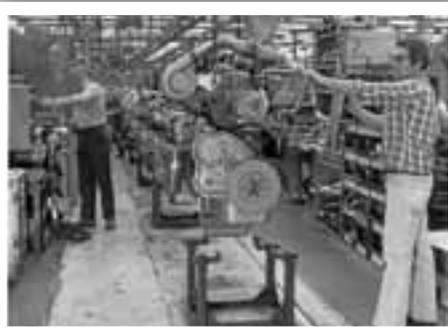
One of the two powered slat conveyors used when the plant opened.
