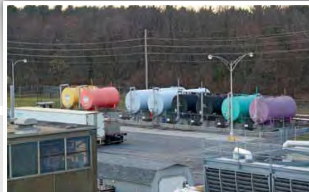
Until 1986, volatile liquids used in production, such as fuels, oils and cleaning fluids, were stored in underground tanks. The tanks were then replaced with safer, more accessible double-walled tanks installed above ground in our enclosed diked tank farm.
